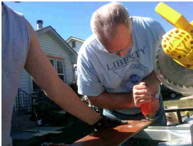
Volunteers working at Rebuilding Together
